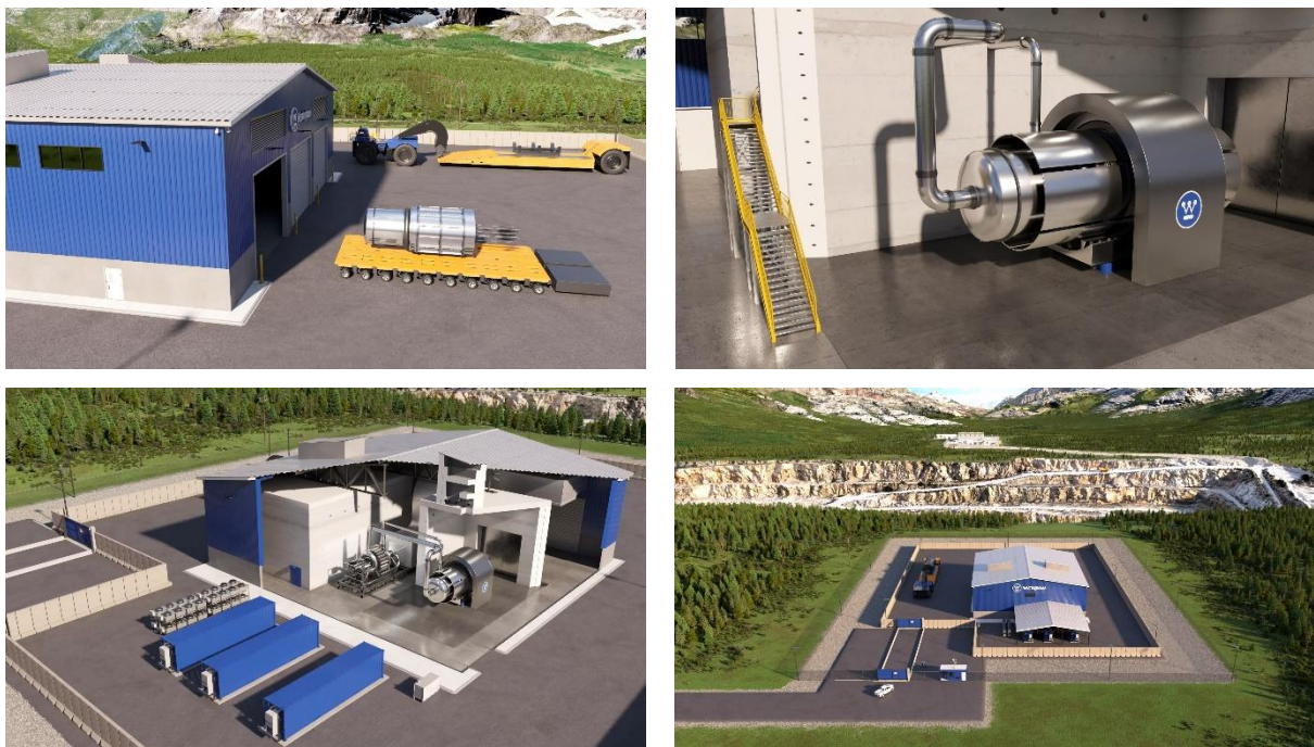
Figure 5 - Computer generated images of the Westinghouse eVinci nuclear micro-reactor representing the installation on a remote site and the easy transportable modular elements
